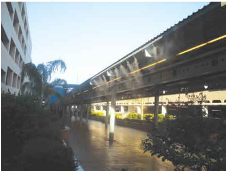
An overhead stream of mist offers Monorail passengers comfort as they travel from the station to the Harrah's and Imperial Palace hotels.
