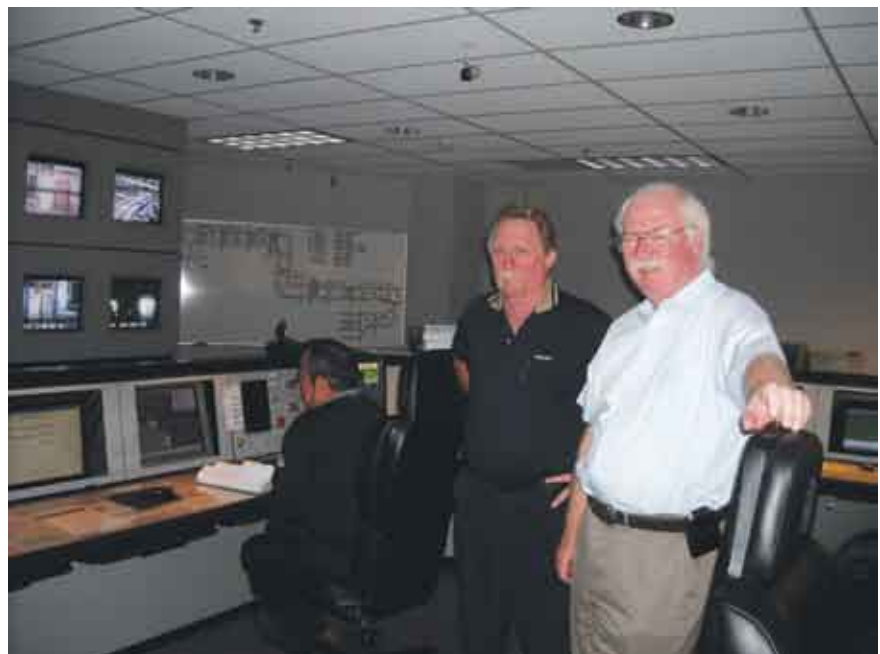
Bombardier's Stephen Stowe (right) and Maintenance Manager Henry Dufresne oversee the Monorail's control center operations, which orchestrates a driverless system providing nearly flawless service.
