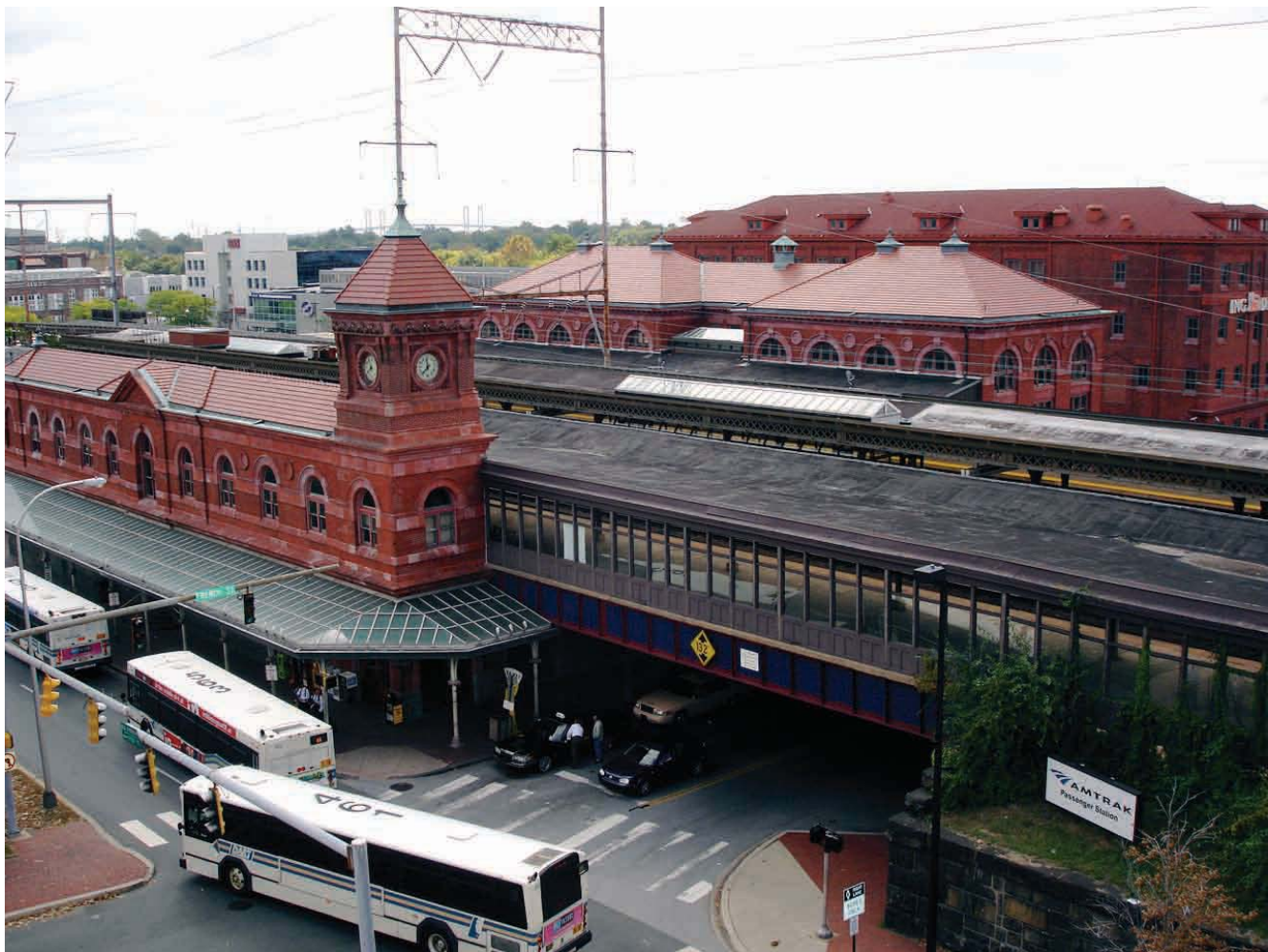
DART buses serve Wilmington Station. The old waiting rooms rise above the tracks on the far side, the structure beyond is Furness' Pennsylvania Building.
