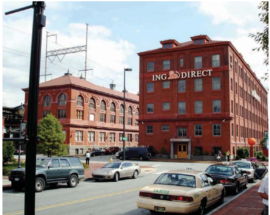
Two of the Furness Buildings: The Pennsylvania Building (right) and the Wilmington Station (left).
